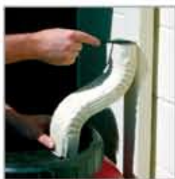
Mark downspout for cutting
