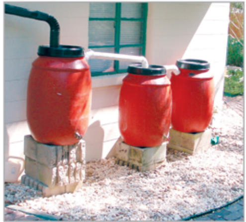
Multiple barrels provide for greater water storage.
