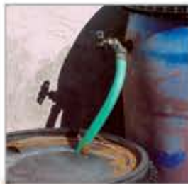
Connecting rain barrels together will allow for more water collection.
